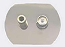
Lubricate rubber seal on largest aperture in eschucheon plate with liquid soap. Slide eschuchen over the 2 valve block stems pushing down evenly and gently in to position, ensuring not to snag and damage the orings on the shower dock stem
