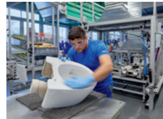
Installation of shower toilets.
