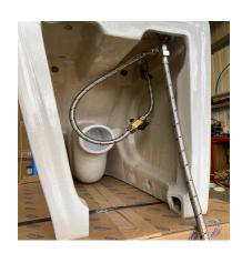
Hidden connection for bottom entry unit with supplied t piece, flexi hose with valve
