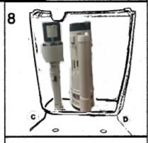
Make sure the inlet flow valve is free from the side of the cistern If the valve is contacting the cistern wall it can not move to close the water and the cistern will continue ti fill with out turning off
